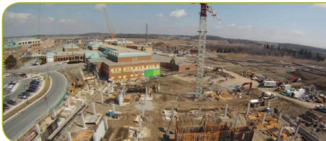
April 2011 – Looking eastward on the Hospital's construction progress
