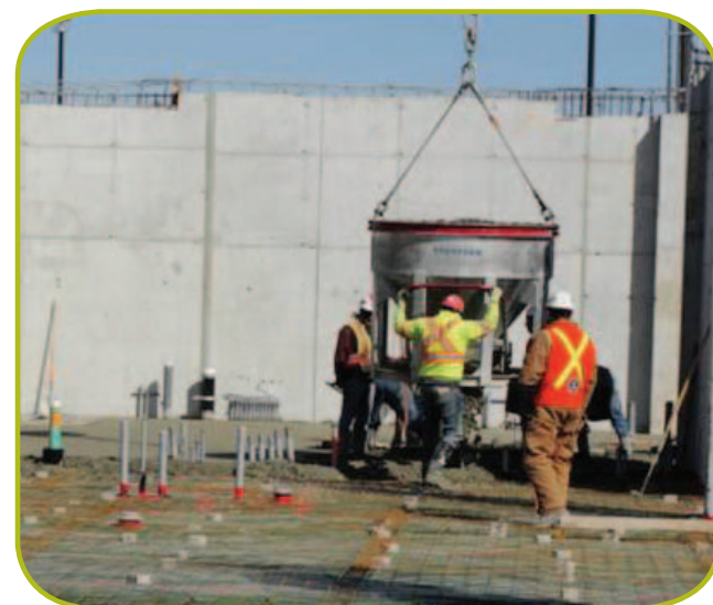
April 2011 – Concrete pour for the new building
