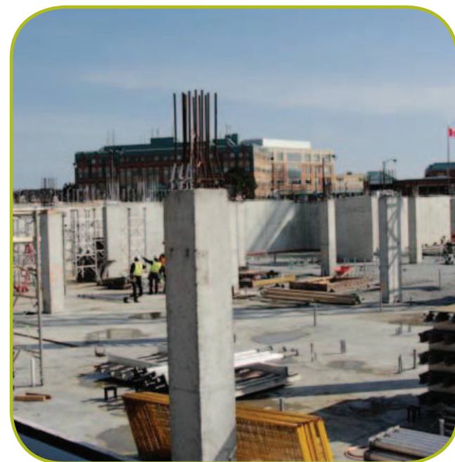
April 2011 – Forming second floor of the new building
